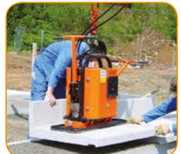
Installation of angled-slabs with Vacu-Magnet 1500 H.
